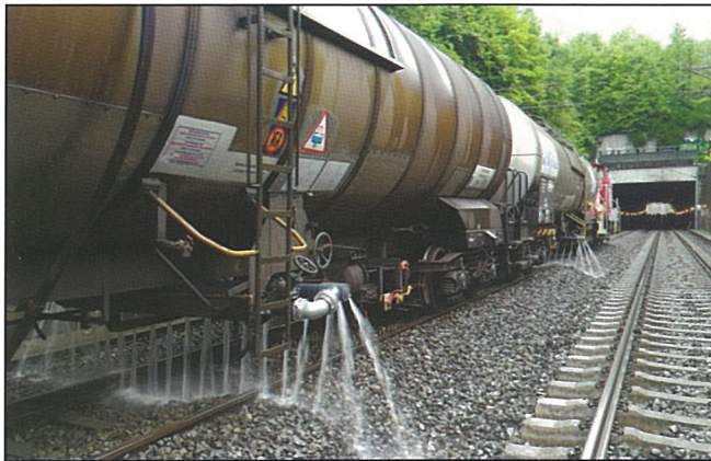
Fig. 4: Ballast being wetted (Photo: Schachner)
