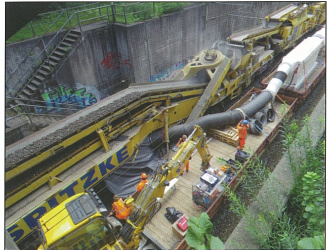
Fig. 5: Vacuuming unit on the adjacent track (Photo: Schachner)
