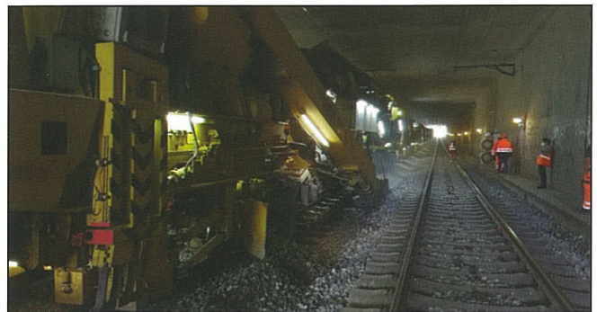
Fig. 6: Minimising dust development during ballast bed cleaning in tunnels (Photo: Schachner)
