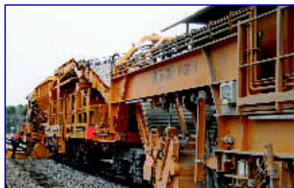
Figure 8: Ballast Distribution System operating in Latvia
