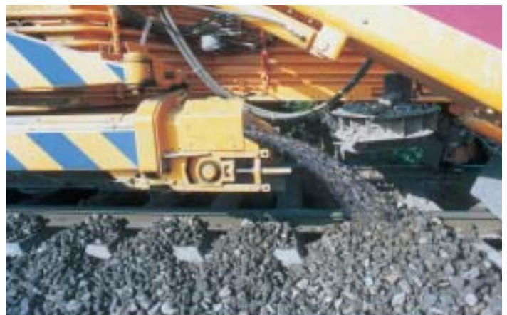
Figure 8: Distributing conveyor belt for re-inserting the cleaned ballast
