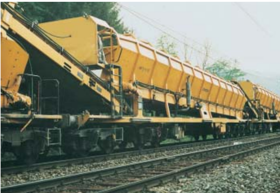
Figure 10: MFS material conveyor and hopper unit for transporting spoil
